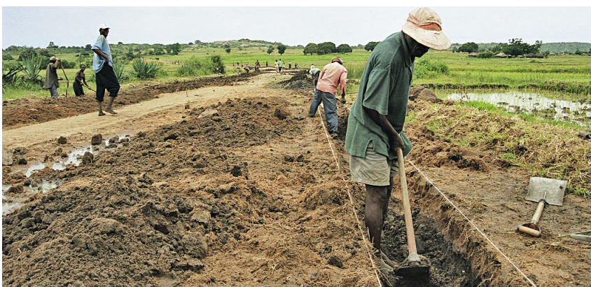
Constructing rural roads in Tanzania
