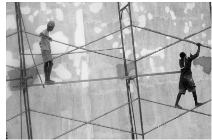
Workers preparing to plaster a wall at 6th floor level on a large building in Dar es Salaam
