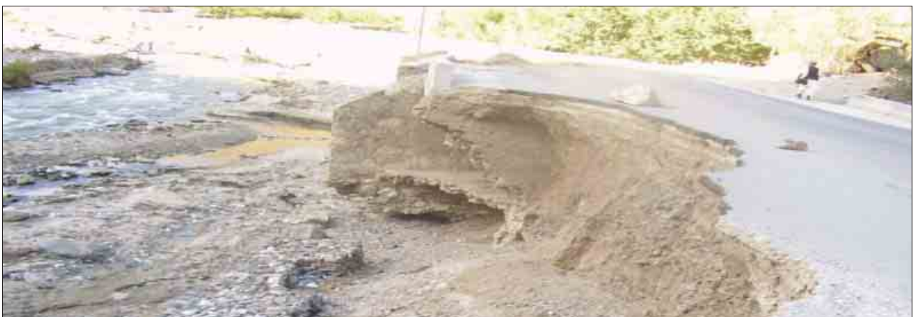
Figure 2b: A section of the highway near Salang damaged by flooding in May 2007.
