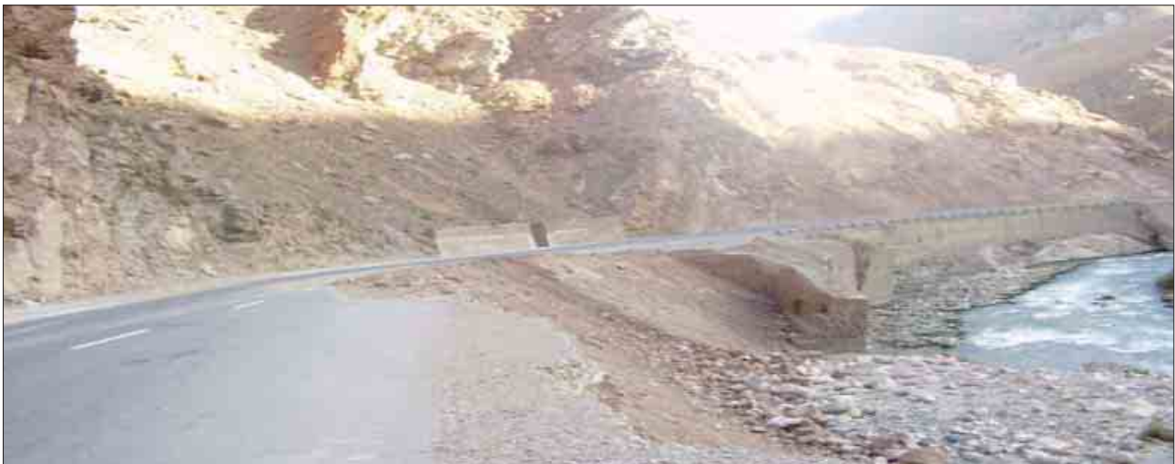
Figure 2a: The highway connecting the north to the capital city, Kabul. The reconstruction of this highway was completed in 2005 but several sections of this road have being severely damaged by flooding after a year due to poor design.
