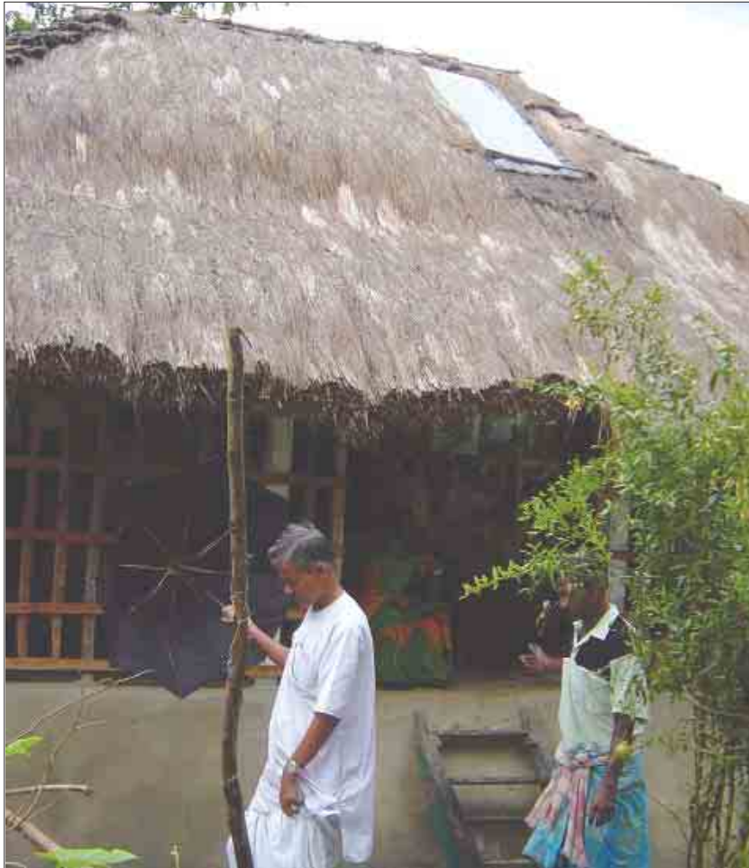
Solar panel, Sunderbans, India
